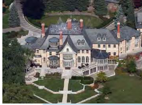
Edgemere 1502 LAKESHORE ROAD E., OAKVILLE, ONTARIO, CANADA
