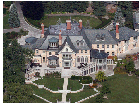
Edgemere 1502 LAKESHORE ROAD E., OAKVILLE, ONTARIO, CANADA
