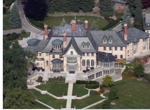
Edgemere 1502 Lakeshore Road E., Oakville, Ontario, Canada
