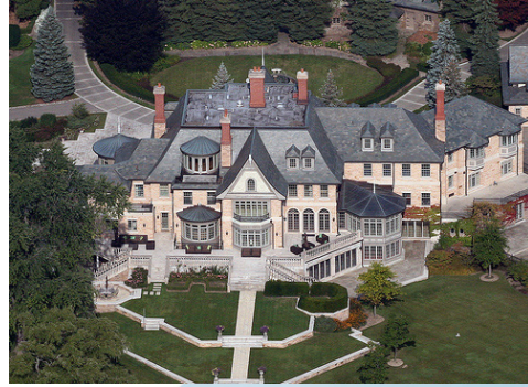
Edgemere 1502 Lakeshore Road E., Oakville, Ontario, Canada
