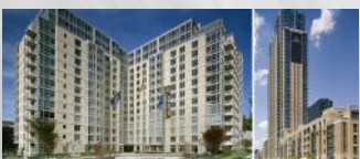
Sheepshead Residential Tower
