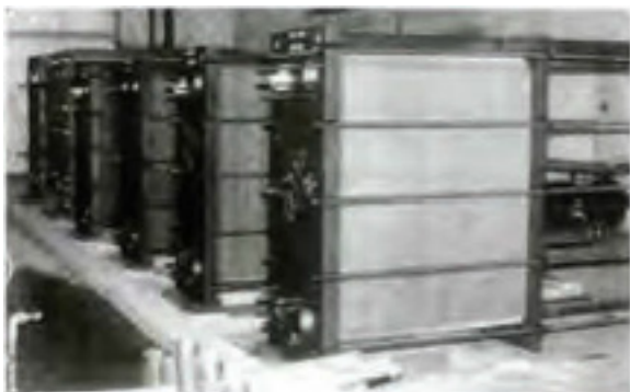
Figure 4.6 Correct position of plates
