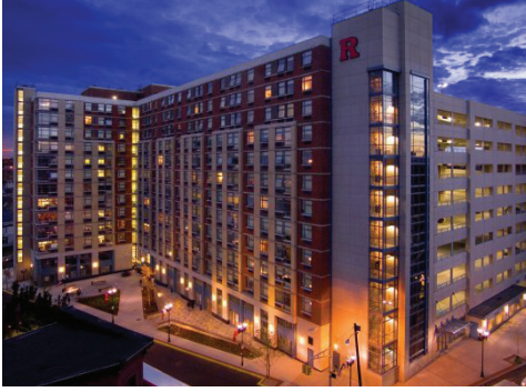
Rutgers University Apartments 604 Bartholomew Road Piscataway, NJ 08854
