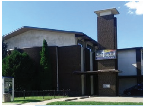
Zion Baptist Church 9802 76 Ave NW, Edmonton, AB
