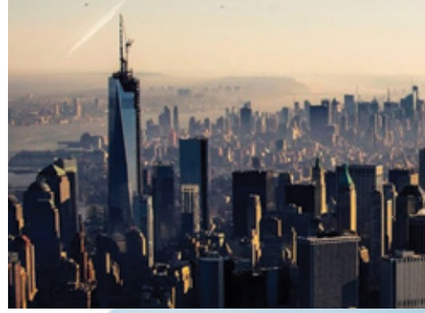
NTT Communications – NTT America 14th floor, 757 3rd Ave, New York, NY, USA 10017
