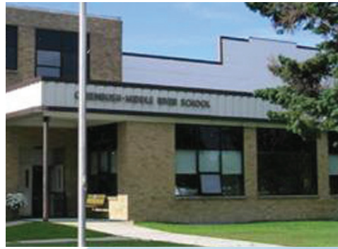
Greenbush Elementary School 127 Greenbush Rd, West Warwick, RI, US
